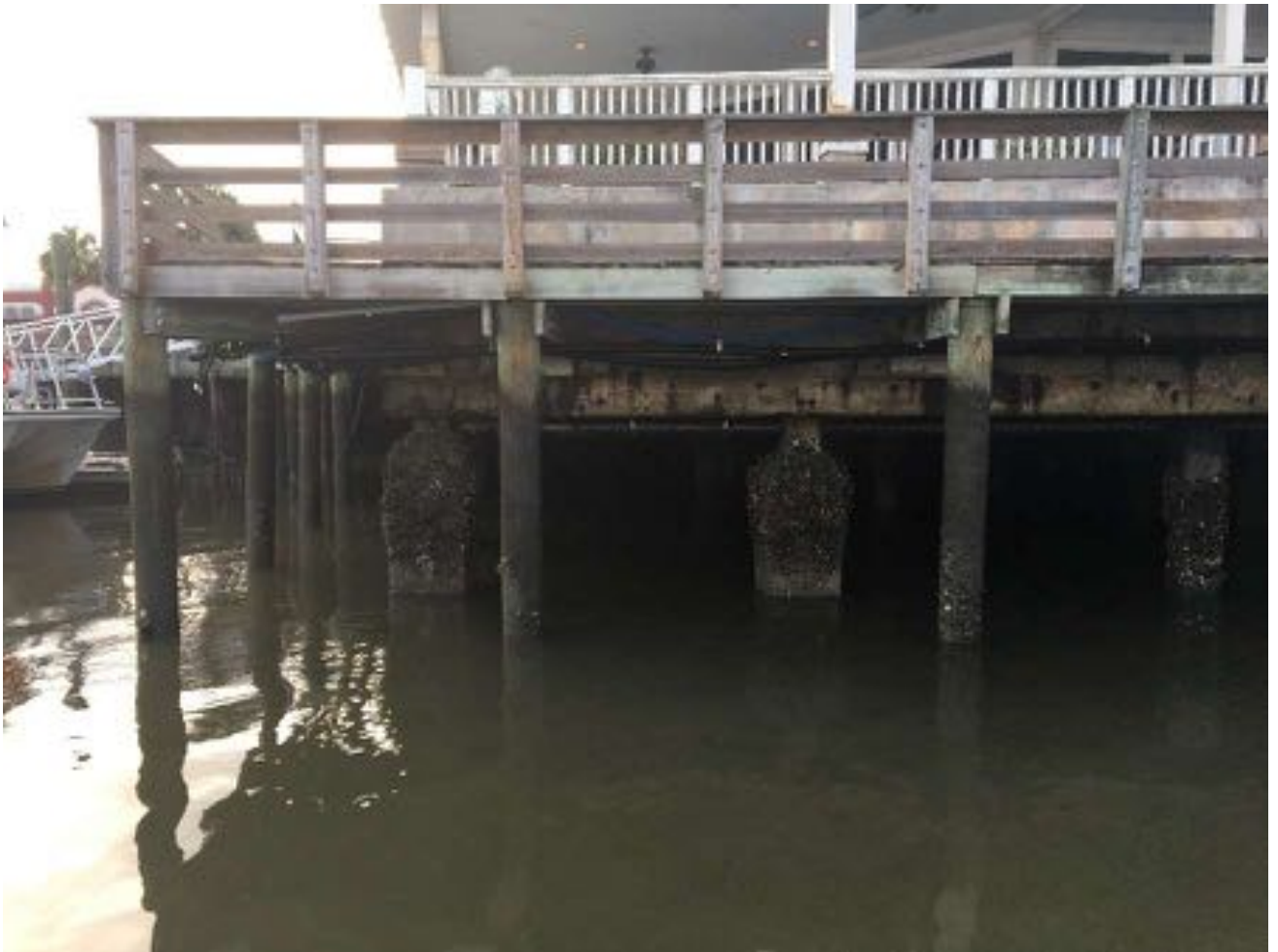
1.01~West Elevation at the Northwest corner of the building
