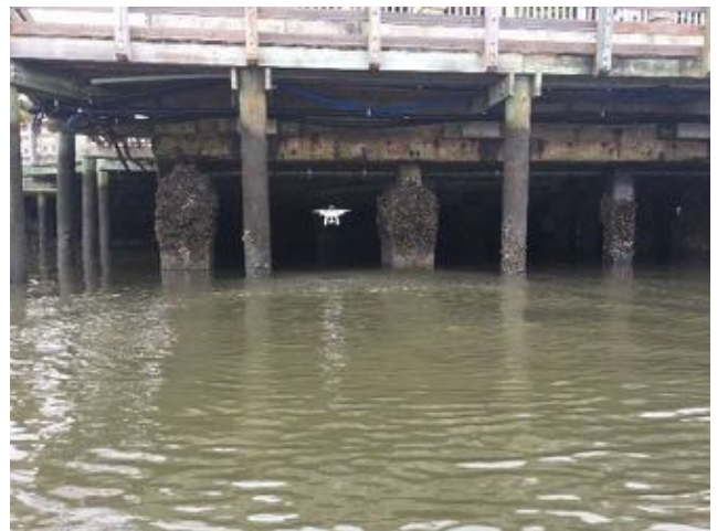
1.18~Aerial drone entering substructure area from the West
